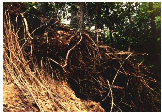
Figure 8. Exposed tree roots in overtopped dam.
